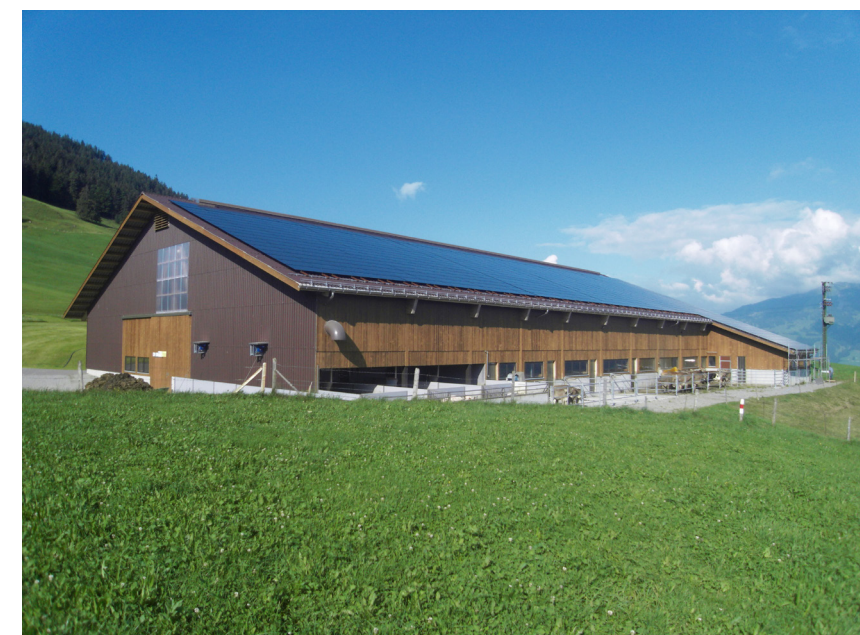
Scheune in Stalden, OW, 125 kWp Photovoltaikanlage (wickisolar.ch)
