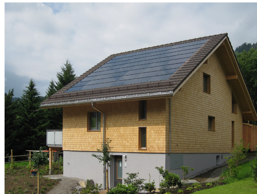
Nullenergie EFH in Flühli, LU, 7.1 kWp Photovoltaikanlage (wickisolar.ch)
